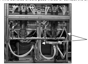
been modified. Wiring has been rerouted and secured along the sides of each unit, away from the springs.
